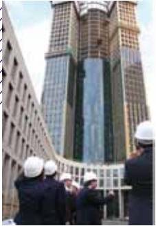
Construction site visit Tower 185
